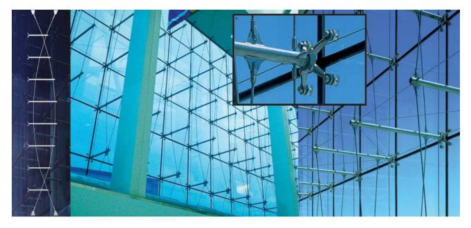
Fig.3: A series of inverted cable trusses define this glass façade. The spreader struts are the only compression elements in the system. Truss stability is achieved by prestressing the cables against the top and bottom boundary supports.<sup>5</sup>
