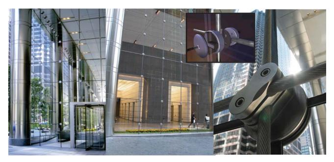
Fig.4: Cable nets top the transparency chart. Here a four-part cast stainless component clamps the cables of this flat 2way flat cable net and clamps the glass to the net.<sup>6</sup>
