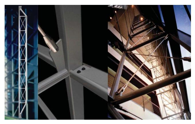
Fig.1: A simple truss system with tension rod bracing and a horizontal purlin mirroring the exterior glazing grid can provide relatively high transparency with considerable economy over more complex truss systems. Virtually any glass system can be adapted to this truss system.<sup>1</sup>
