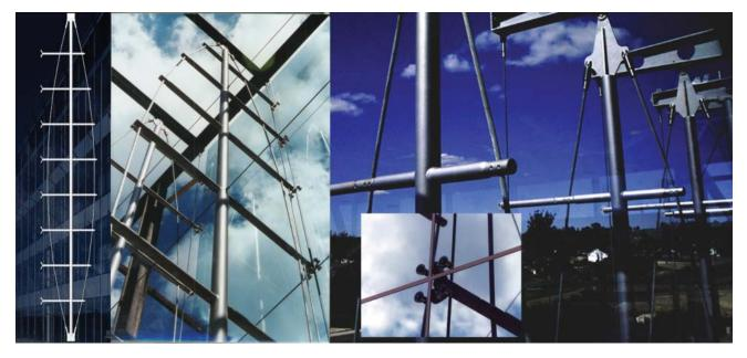
Fig.2: Monolithic glass panes are being attached to the spreaders of these mast trusses. A vertical dead-load cable supports the spreader struts just behind the glazing plane. In this case, horizontal glass will be installed at the top of the trusses back to the building roof.<sup>4</sup>
