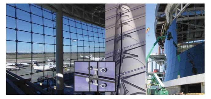
Fig.5: Insulated glass units are point-fixed to this double-curved cable net structure at Sea-Tac International Airport in Seattle.<sup>7</sup>
